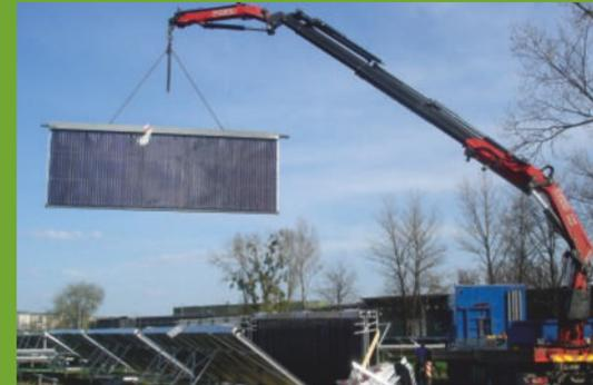
*Structure of the MEGA collector segments with 78 tubes for a large solar collector field*
